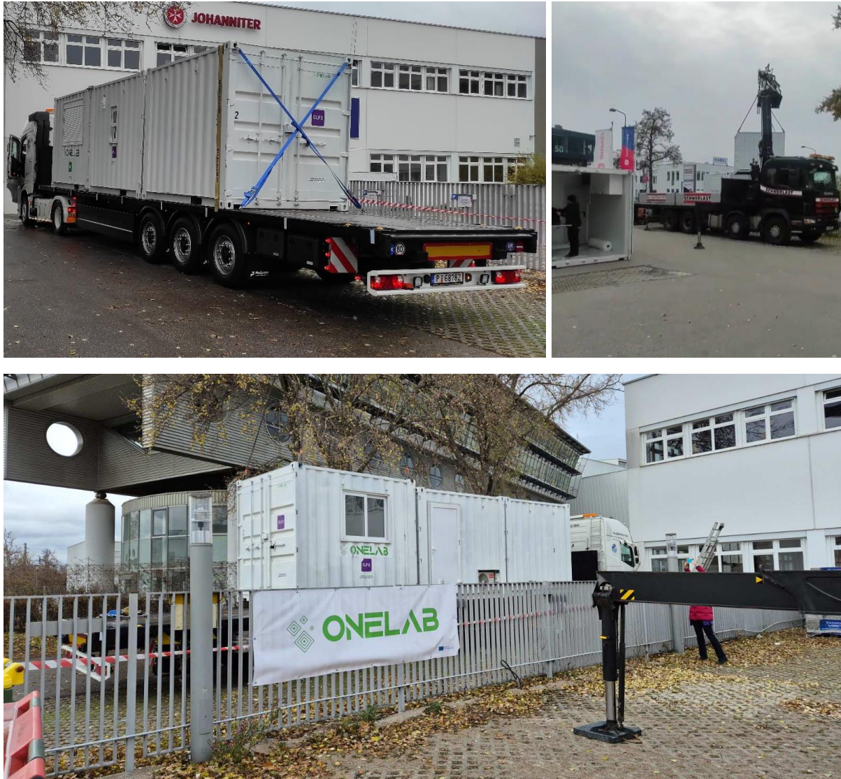
Figure 33 Transportation of the RRML Modules
